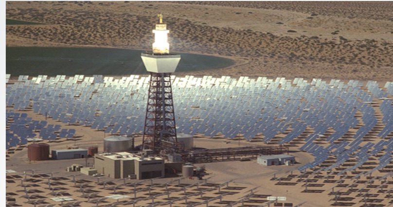
Source: Solar Two, DoE
