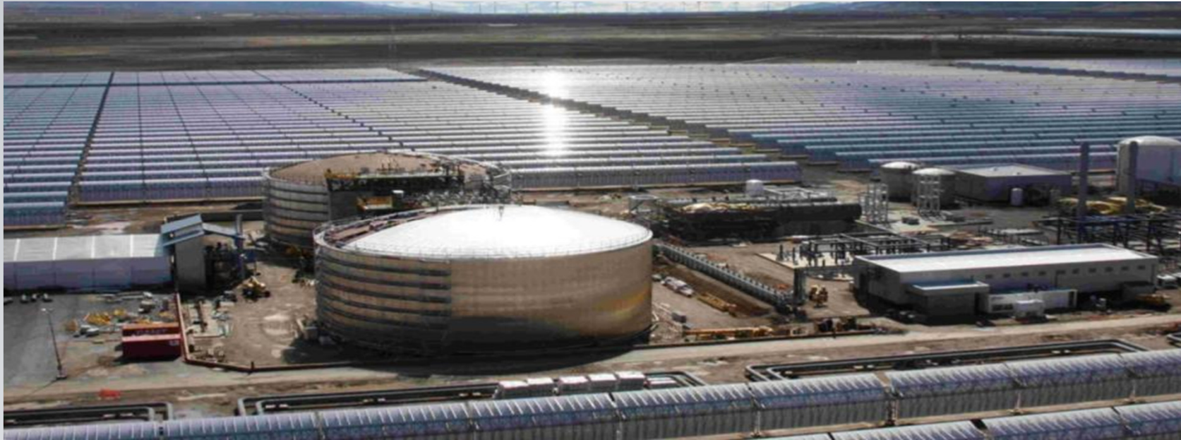
Heat storage tank with molten salt (50 MW | 7,5h)
